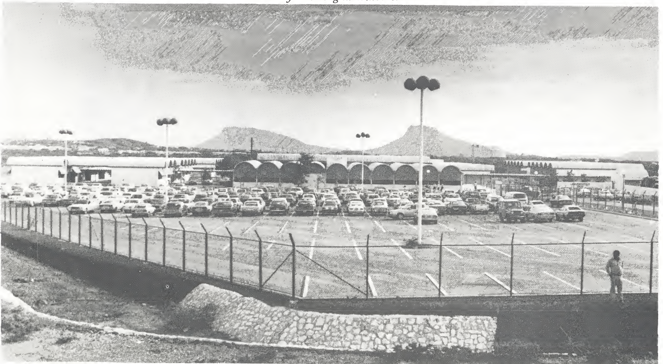
University building in Willemstad
